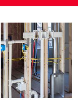
3 Solvent cement the drainpipe to the box hub using approved Oatey primer and cement.
