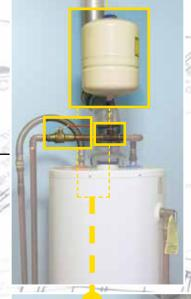
Replace the expansion tank, dielectric union, shutoff valve, and tee with one device!
