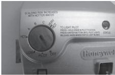
Rotate knob counter-clockwise to the "OFF" position
