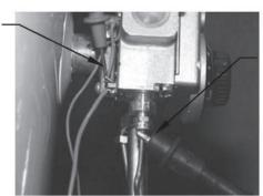
Alligator clip to copper sheath of thermocouple
